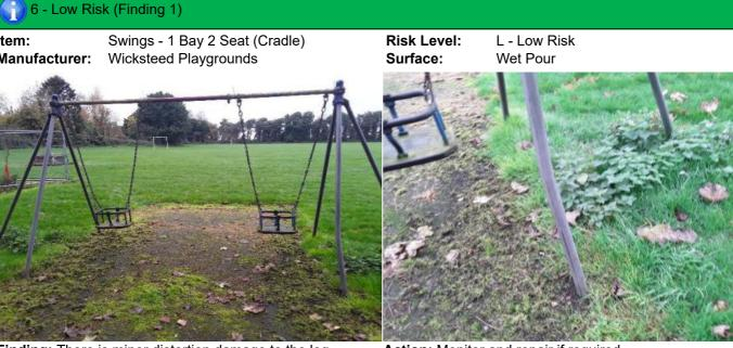
Finding: There is minor distortion damage to the leg Action: Monitor and repair if required
