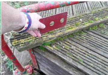
Finding: The item fails to meet the requirements of BS EN Action: Monitor - No remedial work recommended 1176 Part 1 4.2.7.2 for head and neck entrapment in the handgrip openings
