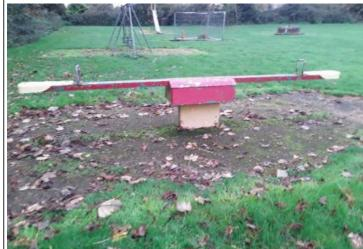
**Finding:** The item fails to meet the requirements of BS EN 1176 Part 1 4.2.7.2 for head and neck entrapment in the handgrip openings
