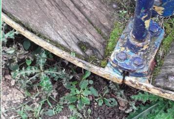
**Finding:** There are parts of the timber around the fixing points that have rotted
