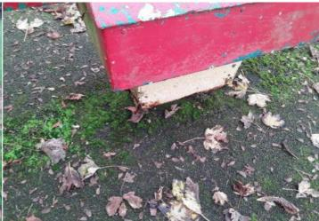
**Finding:** There is no gaiter protection for accessible moving **Action:** Monitor - No remedial work recommended parts (possible shear trap) as recommended in BS EN 1176 Part 1; 4.2.6 Moving Parts
