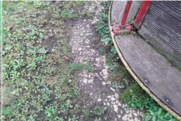
**Finding:** The safety surface has degraded / reduced and the concrete foundations are exposed
