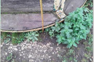
**Finding:** The distance between the underside of the roundabout platform and the playing surface is in excess of 110mm and contravenes the requirements of BS EN 1176 Part 5 which requires that the distance be maintained between 60mm-110mm - for the entire circumference of the roundabout
