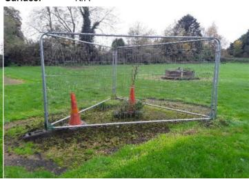
Finding: A redundant damaged area of wet pour has been Action: Consider reinstating the area to grass fenced off preventing access
