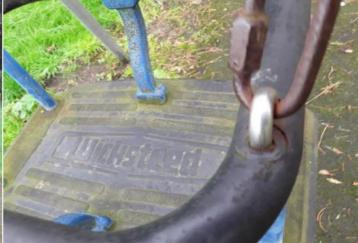
Finding: The swing seat frames are corroding
