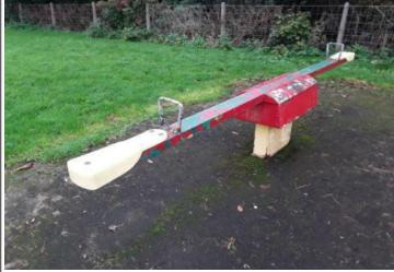
Finding: The pivot mechanism is showing signs of wear
