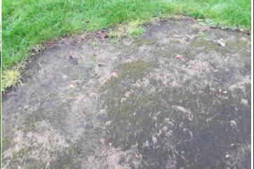
**Finding:** There is algae, silt or moss growth on the surface **Action:** Clean and treat appropriately resulting in slippery conditions
