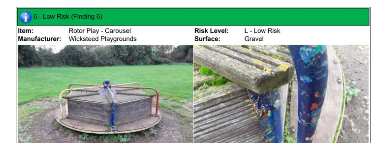
Finding: The paintwork on this item has been damaged or Action: Treat affected areas and repaint worn exposing the metal underneath which is rusting / corroding
