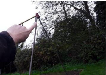
Finding: One of the lateral frame stabilisers is missing
