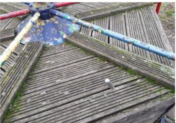
**Finding:** There is/are finger entrapment/s in the structure and the item fails to meet the requirements of BS EN 1176 Part 1 4.2.7.6 Entrapment of fingers
