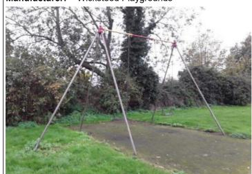
Finding: There are excessive chain tails provided, however Action: Cut back excess chain tails but ensure a minimum a minimum of 2 additional links should always be provided with crucifix connectors
