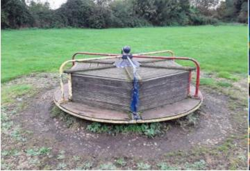
**Finding:** There are areas or parts of the timber on the structure that have rotted around fixing points
