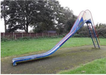
**Finding:** There is/are finger entrapment/s in the framework and the item fails to meet the requirements of BS EN 1176 Part 1 4.2.7.6 Entrapment of fingers
