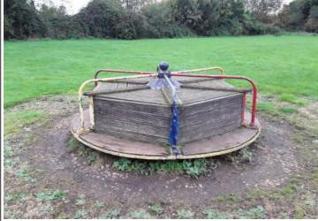
**Finding:** The safety surface has been removed, and in addition, the edge dimensions do not meet with the requirements of the current applicable standard (2.0m impact area required around the item - client notified)
